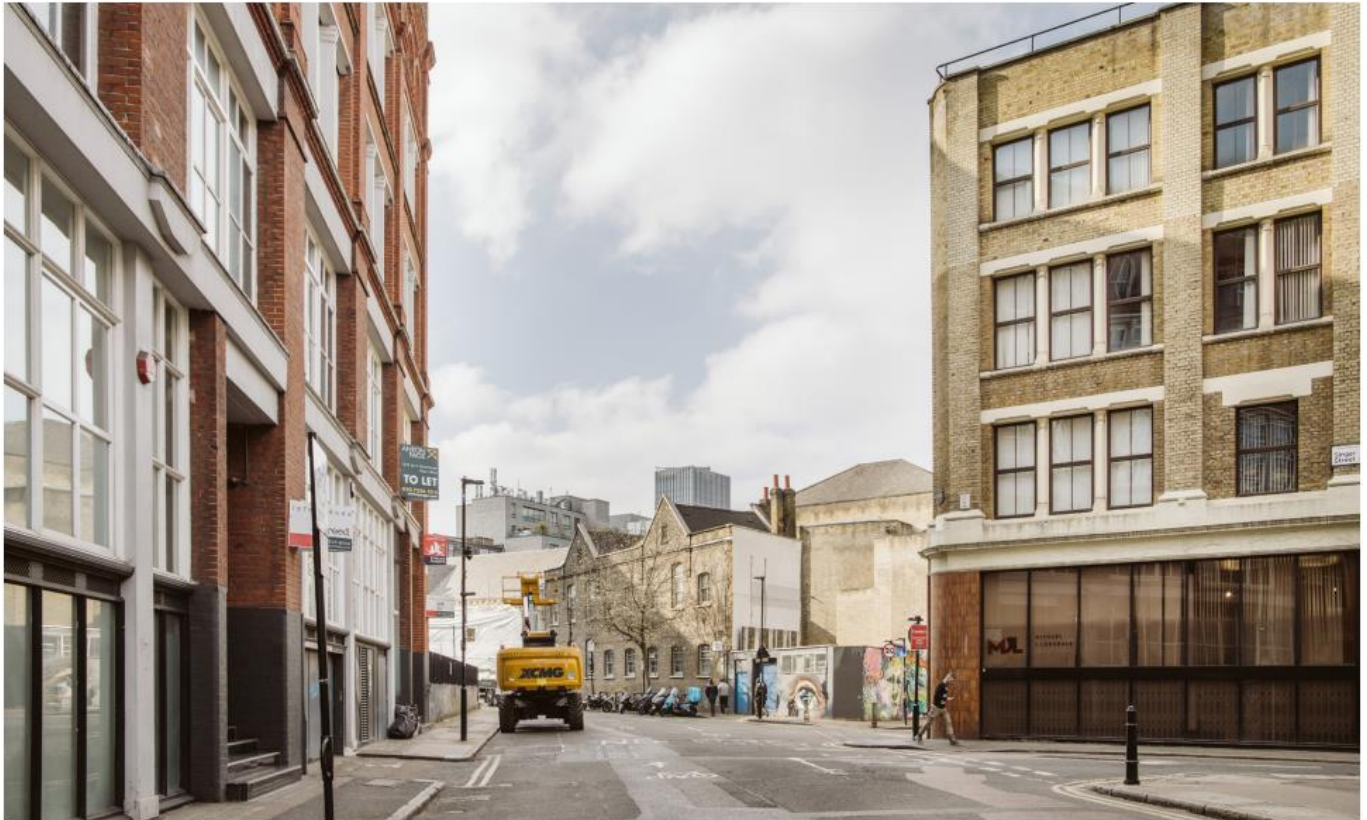
Image 3– View looking south along Tabernacle Street (former sixth form centre seen in centre to be demolished)
