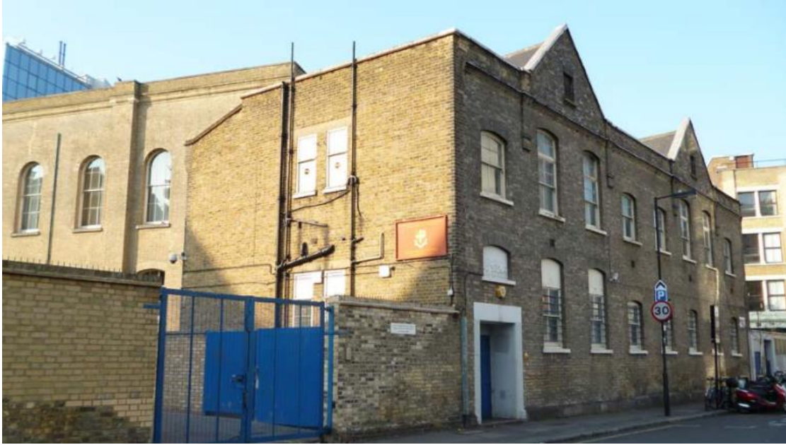
Image 7 – Former Sixth Form Building, the demolition of which was consented via P2017/1046/FUL
